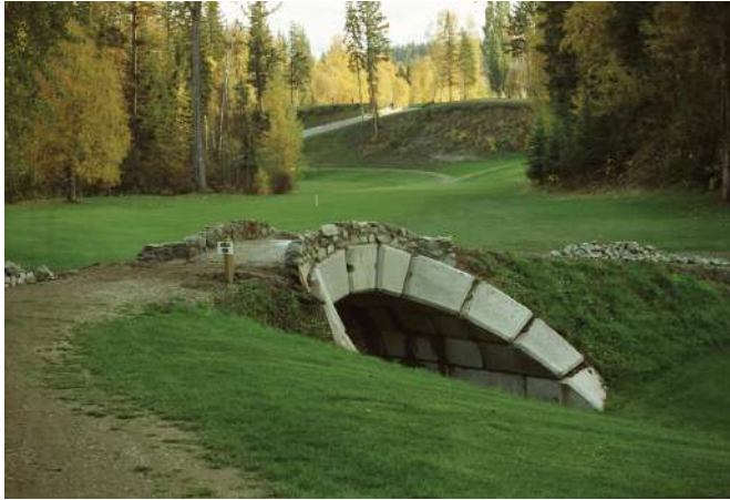
A tapered Arch-Lock™ bridge over a creek
