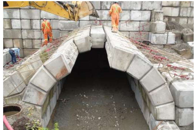
3 Arch-Lock™ structures for a water infiltration vault
