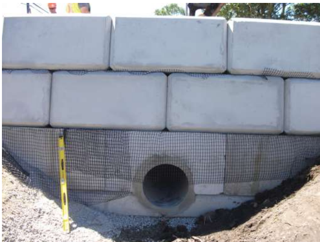
Headwall comprised of Lock-Block™ units with geosynthetic soil reinforcement.
