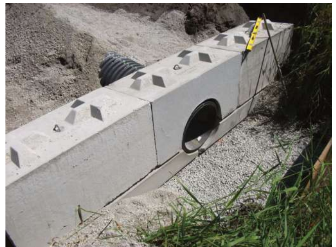
Keyed Two-Cross Lock-Block™ units in headwall
